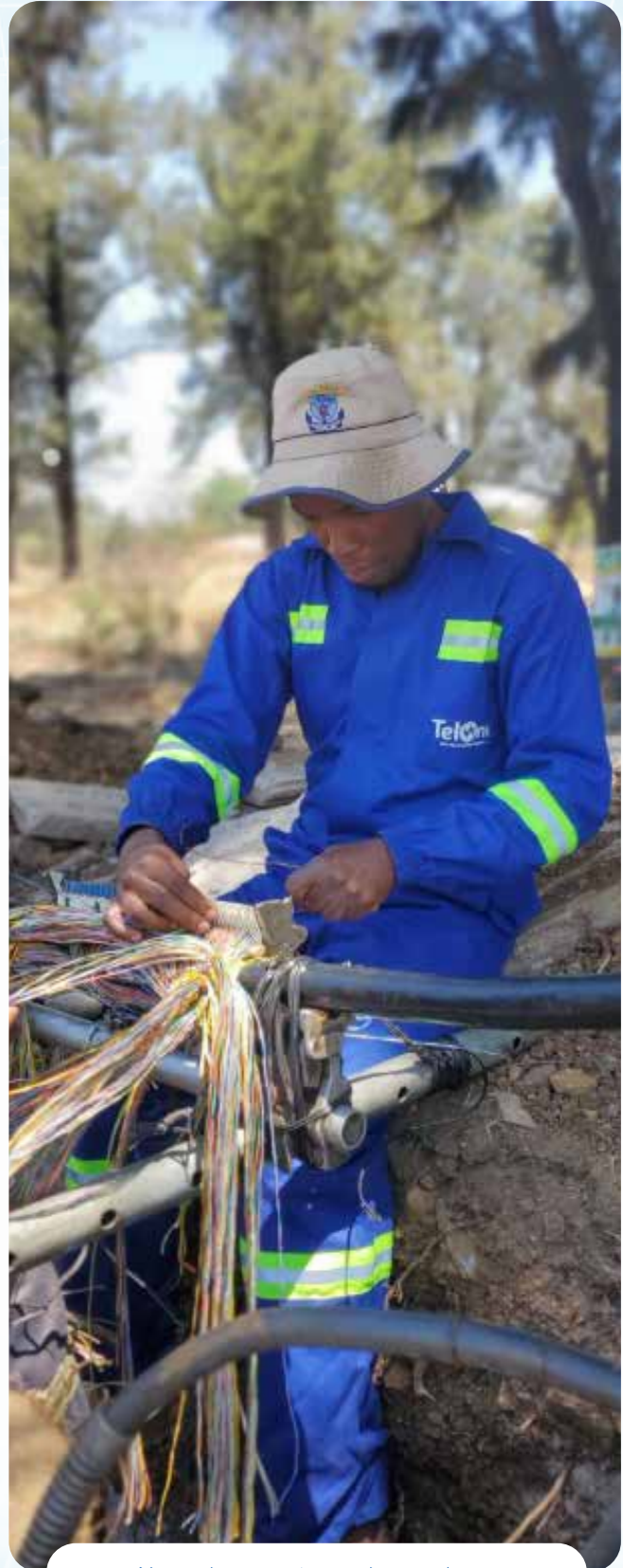
Network expansion and upgrades
