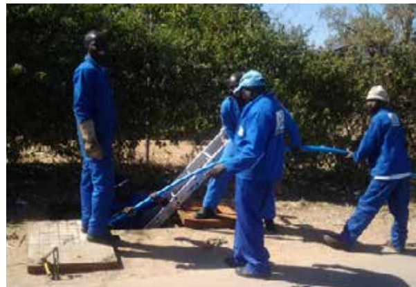
TelOne technical team rolling out fibre
